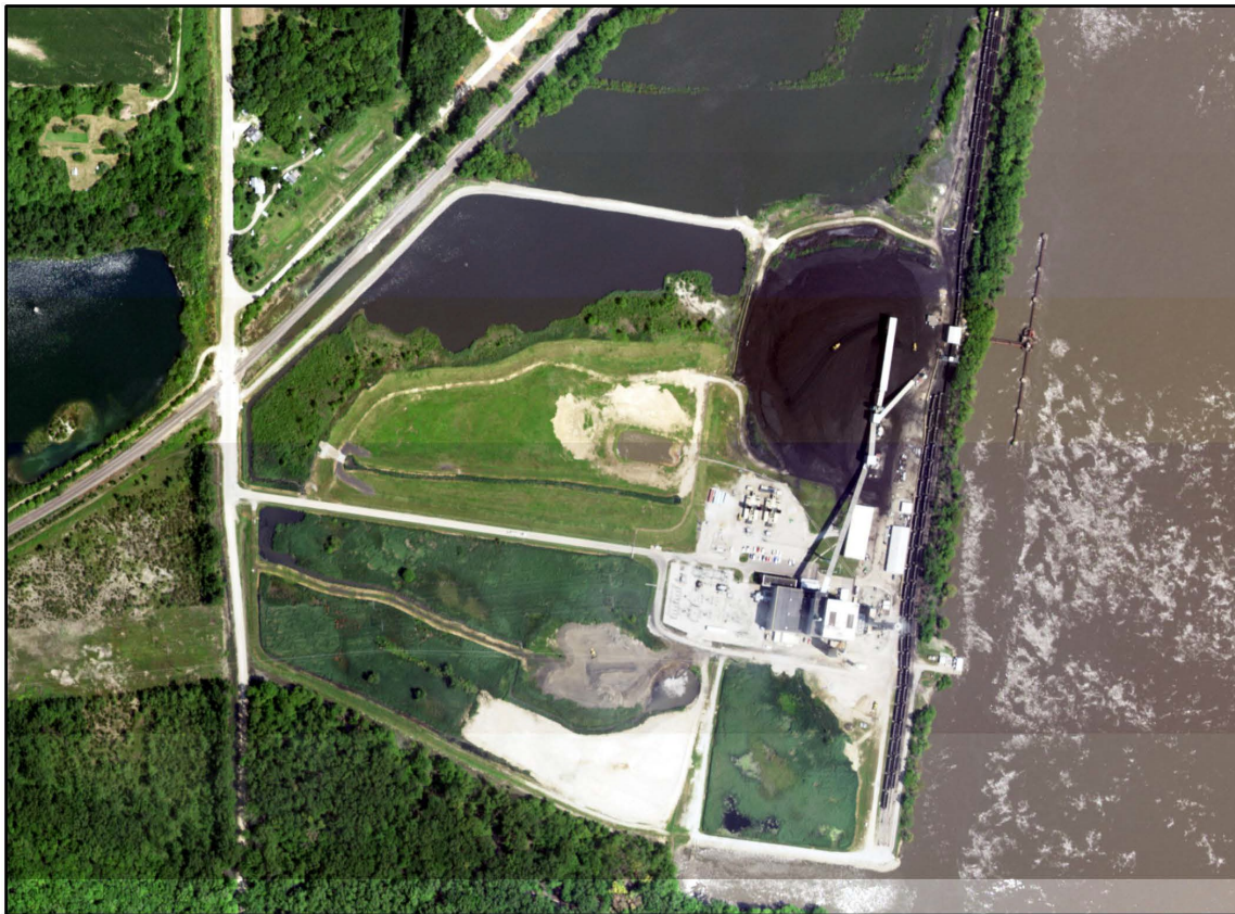
Figure 4.1: Aerial Photograph of the Burlington Generating Station
