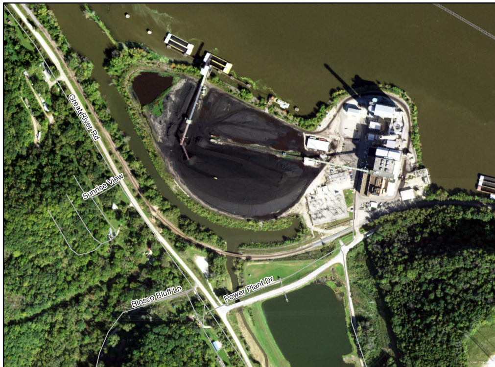
Figure 3.1: Aerial Photograph of the Lansing Generating Station
